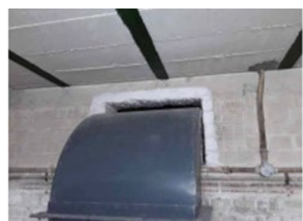
Residue around Air Vent
