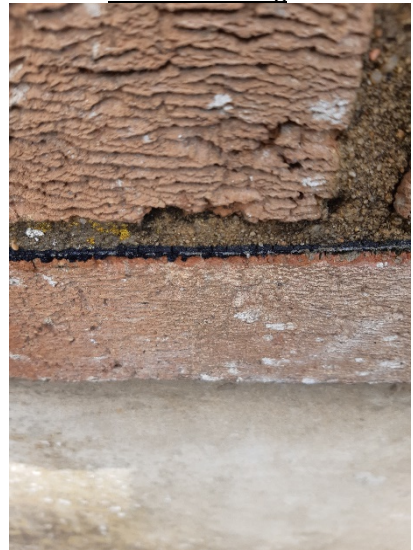
Bitumen Damp Proof Course
