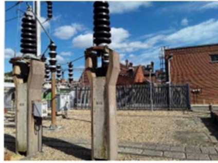
Panels to Concrete Structures
